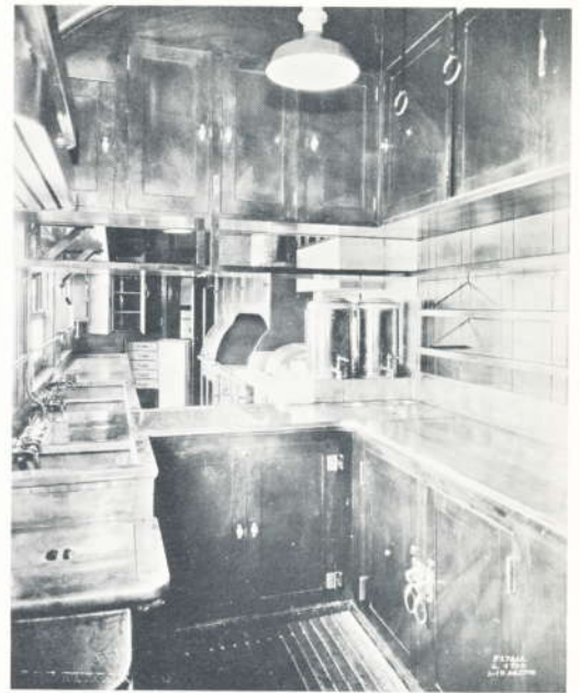
This view is from the pantry with its many food storage lockers — some ice cooled — and the two coffee urns to the right, looking into the kitchen. They had electric lighting throughout and were considered the finest Diners in operation.
