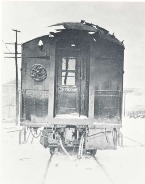
This is the Dummy End of SP 10098, a 77-D-3 class Diner. Both classes were equipped with National Malleable Type "D" head couplers and 6-wheel trucks equipped with Westinghouse type U.C. brake system.
