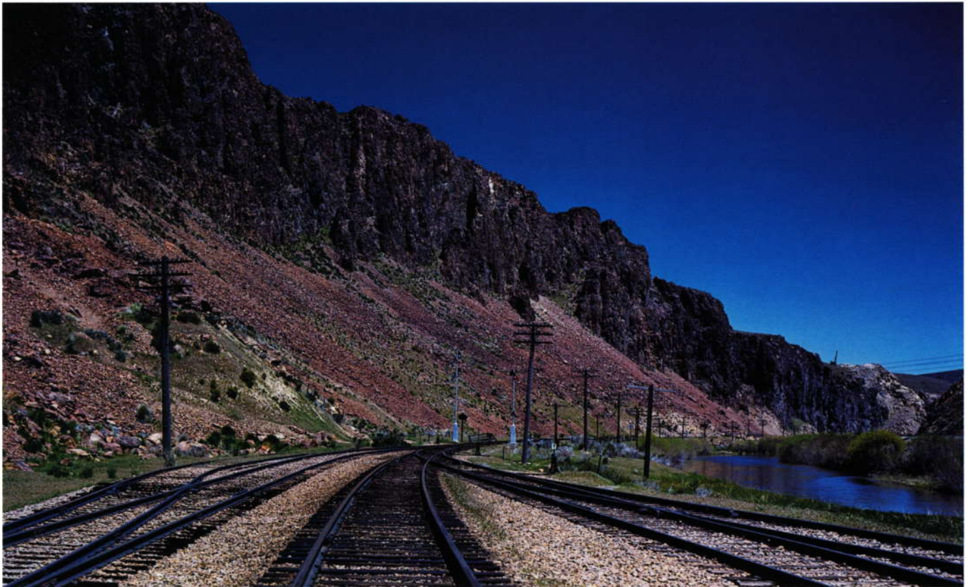
Though SP's trackage through Nevada traverses many wide, flat valleys, there are rugged portions of the line. This is one of them, alongside the Humboldt River in Palisade Canyon, located in eastern Nevada. Semaphore signals still guard the track in this view.
